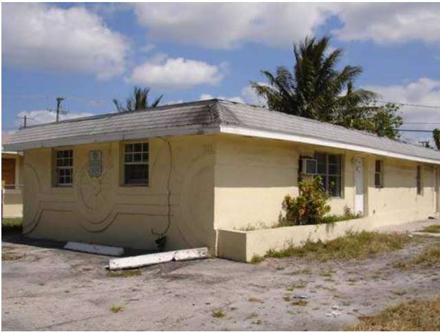
Figure 15: Lack of maintenance
