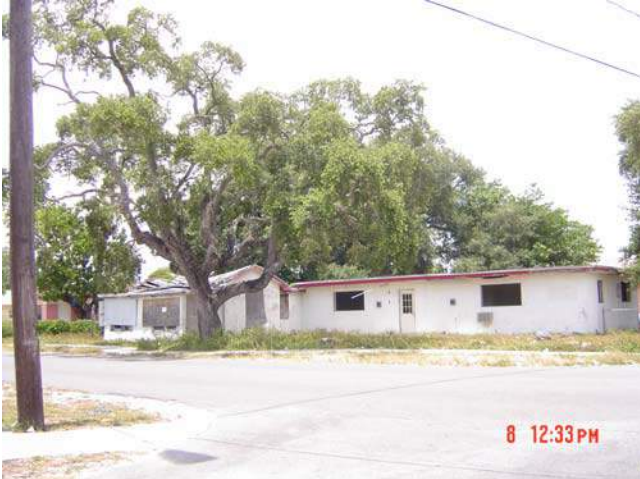
Figure 24: Abandoned, dilapidated structures
