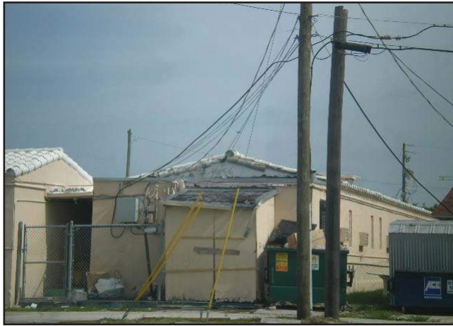
View of commercial rear from street; needs beautification
