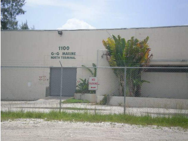
Figure 2: Unpaved parking and pedestrian access
