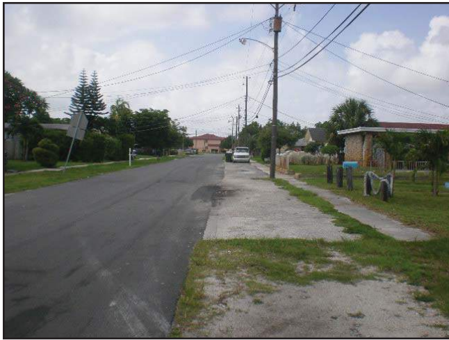
Unfinished infrastructure lacking swale and sidewalk maintenance
