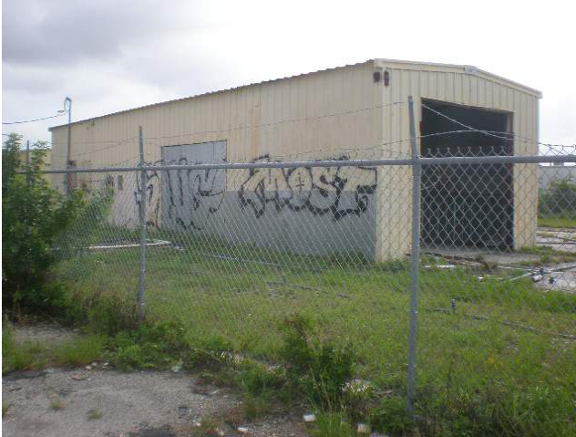
Figure 28: Abandoned structure, vandalized
