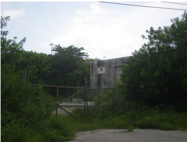
Figure 1: Overgrown and deteriorated site - unsanitary and unsafe conditions
