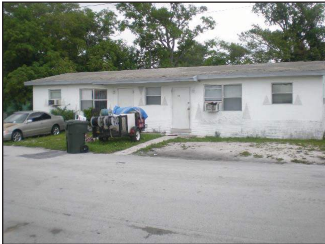
Deteriorating structure and site conditions – inadequate parking
