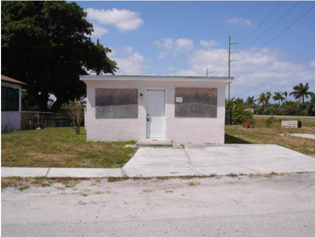
Figure 18: Vacant unit with boarded windows
