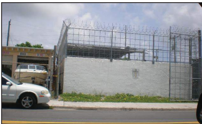
View of businesses from street; needs beautification
