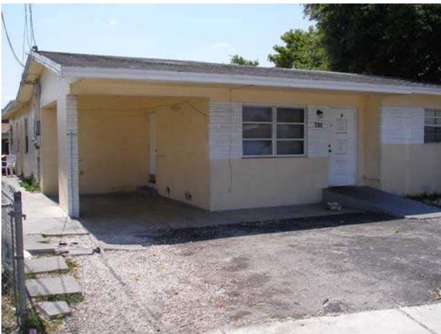
Figure 13: No landscaping, lack of site maintenance
