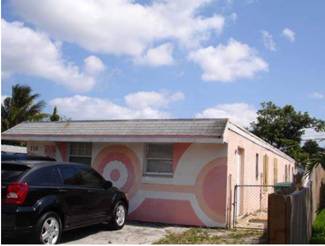
Figure 11: Multi-family with boarded windows
