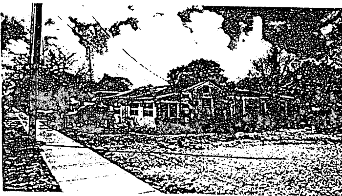
Photograph 3 Single family home in poor condition on NW 5 th Avenue and 3 rd Place.
